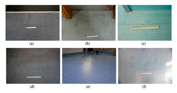
**Figure 4.** Anomalies: (**a**) A-A1 scratches; (**b**) A-A1 wear; (**c**) A-A3 brightness changes; (**d**) A-A3 brightness changes on a linoleum flooring due to an inadequate maintenance; (**e**) A-B2 peeling, requiring the use of repair technique R-B2 partial replacement; (**f**) A-B3 depression/settlement, requiring the use of repair technique R-B1 total replacement.
