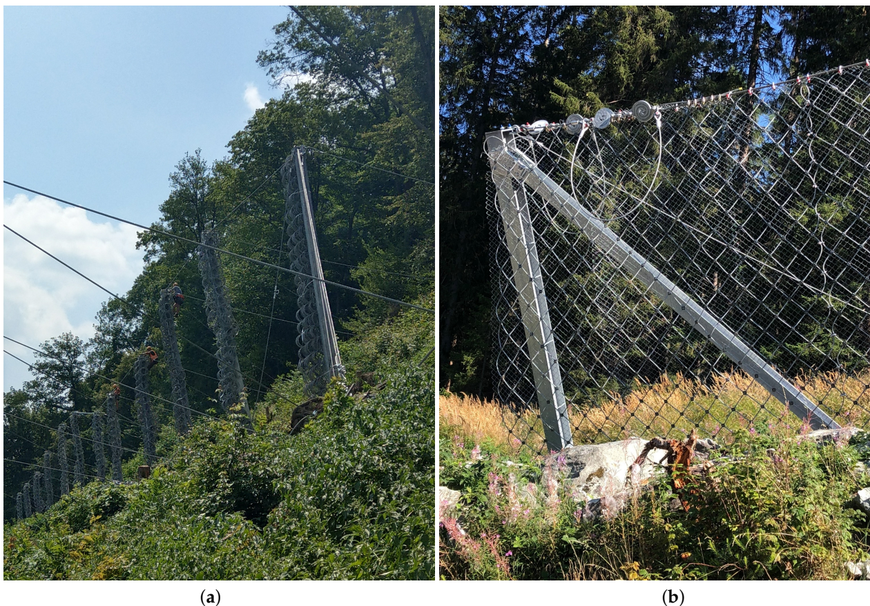
Figure 1. (a) Installed posts with pre-installed net panels according to clear and easy to implement mounting instructions; (b) modification at the lateral end of a barrier without lateral anchors with a diagonal strut as replacement.
