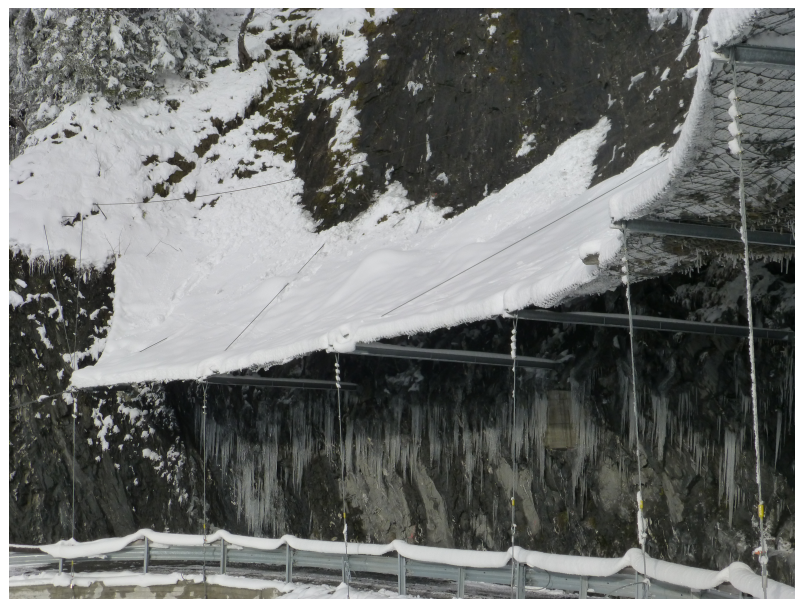
Figure 3. Rockfall protection barrier suffering from snow load.
