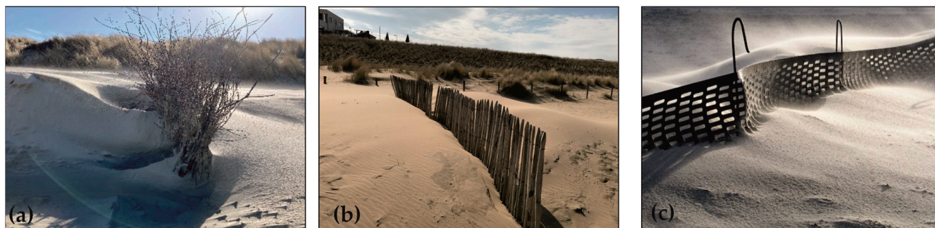
Figure 2. Examples of different design types of sand trapping fences: (a) brushwood, (b) vertical plank, (c) perforated plastic. Photograph in (c) is published with permission from Peter Tigges [42].
