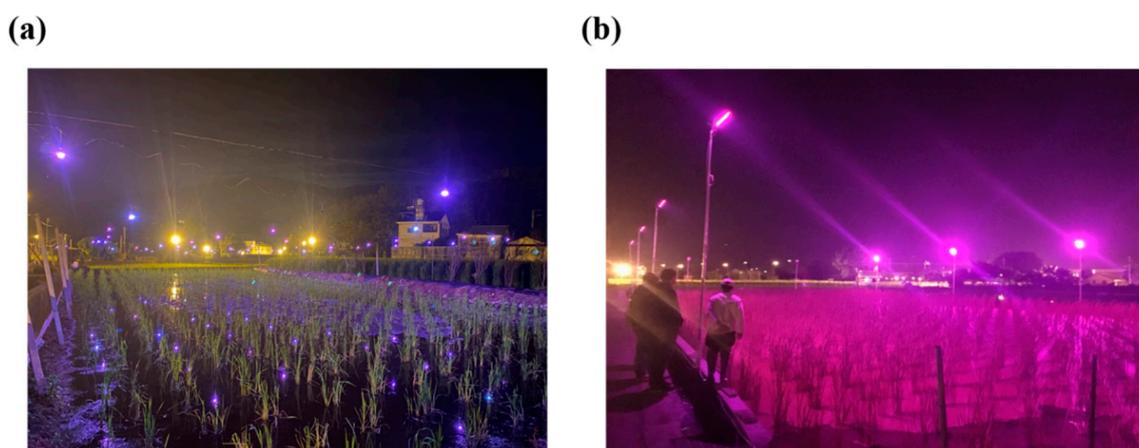
**Figure 1.** (a) A light emitting diode (LED) lamp-integrated agriculture facility constructed by the Industrial Technology Research Institute (ITRI) team in Taiwan. Each LED lamp is hanging above the water bamboo leaves. (b) An LED array module lighting lamp, with blue and red LED bulbs constructed near the ridge in an array format.
