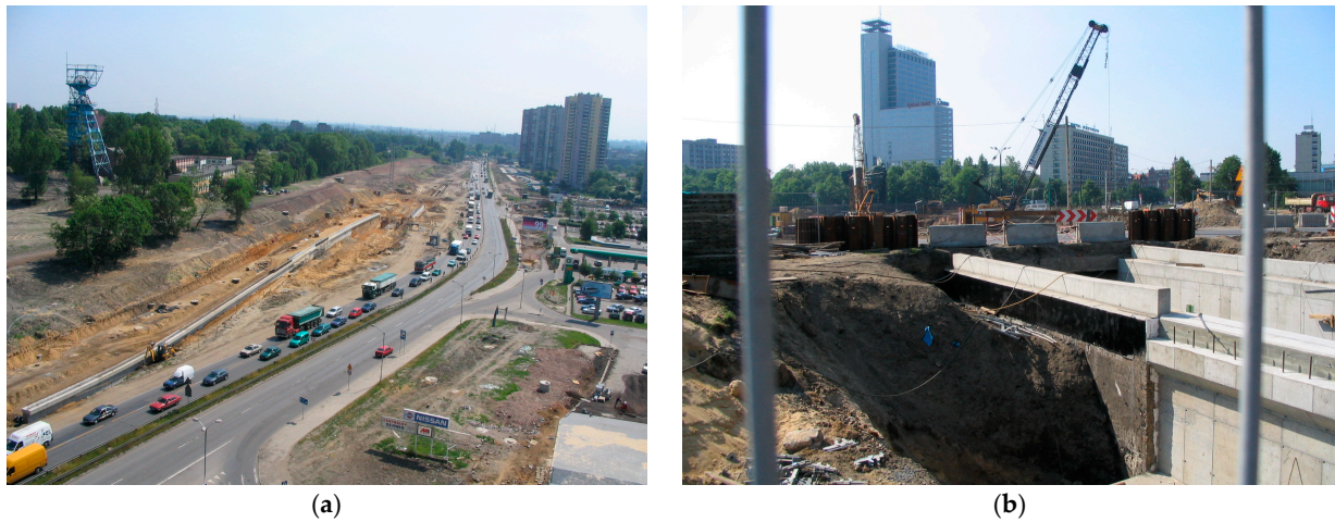
Figure 7. Execution of works as part of the construction of the tunnel under the Roundabout in Katowice: (a) beginning of the tunnel; (b) construction of diaphragm walls.
