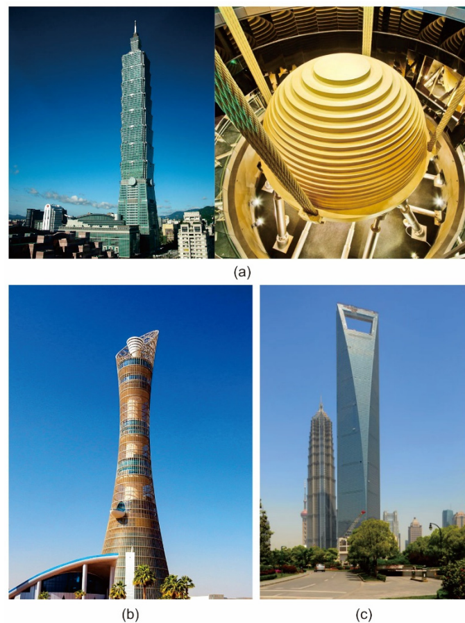
Figure 2. Tuned mass damper applications: (a) 101-Taipei, Taipei—Taiwan; (b) Aspire Tower, Doha—Qatar; (c) Shanghai World Financial Center, Shanghai—China.
