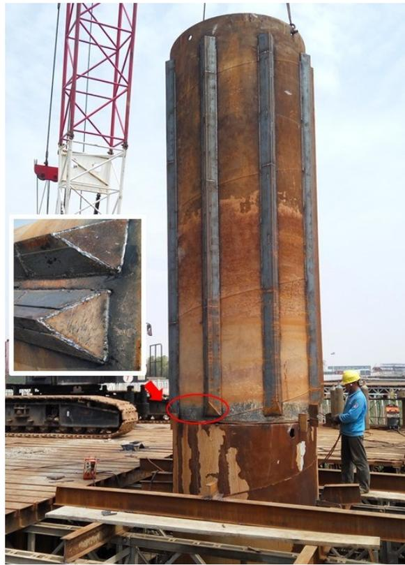
**Figure 2.** Angle steel outside the steel casing.
