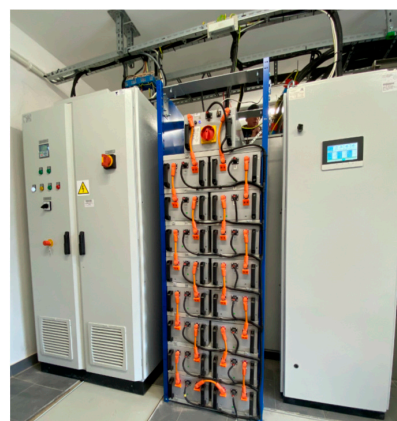
Figure 8. A prototype of a 100 kW energy storage system using LTO technology.
