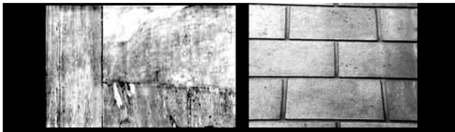
**Figure 16.** White Pentelic marble surface (left) and Kapandriti's stone surface (right) at the historic Bank of Greece building in Athens.
