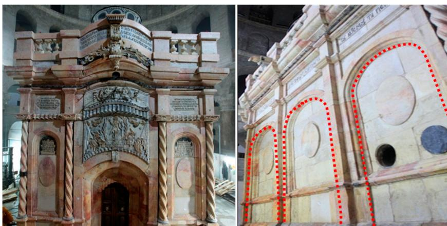
**Figure 35.** East façade (entrance) of the Holy Aedicule (**left**); façade areas where the stones were removed and then reassembled (**right**).
