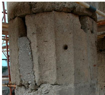
**Figure 27.** Concrete and cement products were used to fill the drums.
