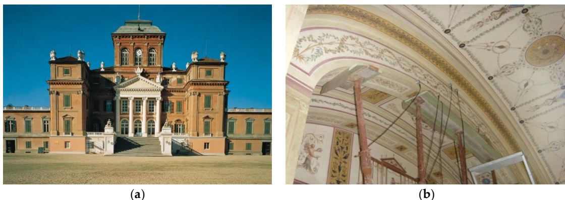
Figure 14. External view of the Racconigi Castle (Italy) (a) and the monitored masonry arch inside the Castle (b).
