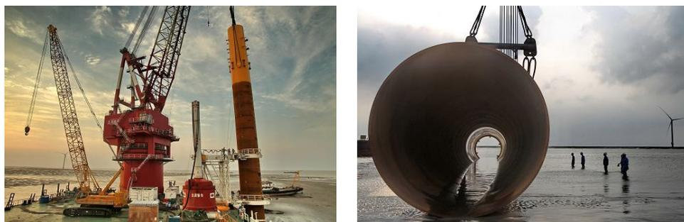
**Figure 2.** Monopile for a 150 MW offshore (intertidal) wind farm in Longyuan, Rudong, Jiangsu.
