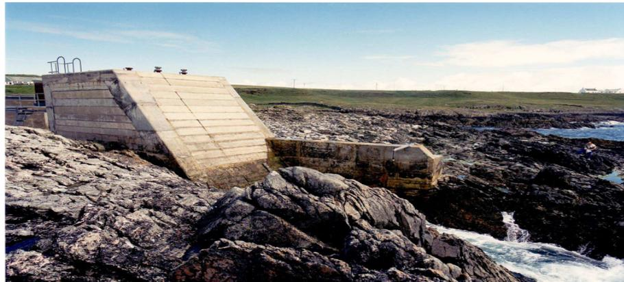
**Figure 3.** Oscillating water column on the island of Islay, Scotland, (courtesy of M. Folley).
