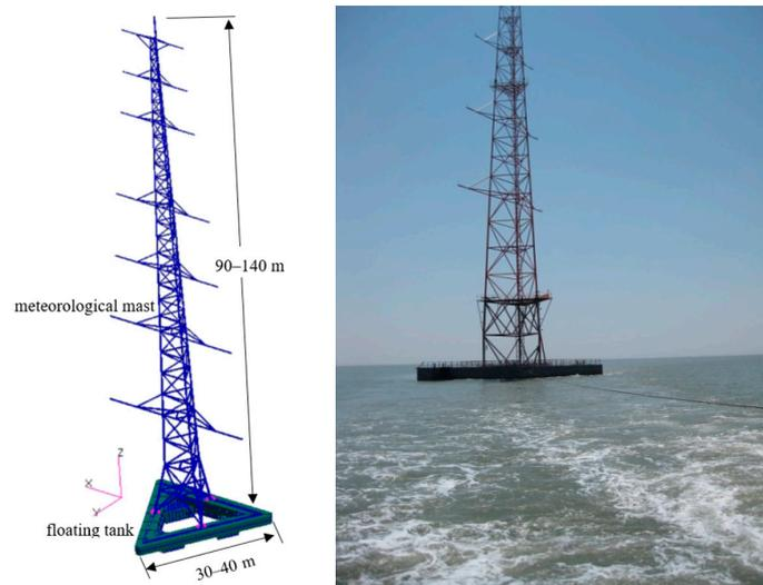
**Figure 1.** Offshore integrated meteorological mast and towing operation.
