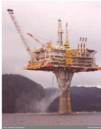
**Figure 1.** The Draugen platform ready to be towed to site in 1993. Note the slender concrete shaft and the widening at the top to support the topside facilities.
