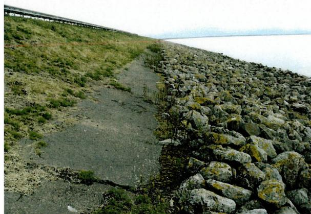
**Figure 1.** Rock armour on the low part of the seaward slope (from [12]).
