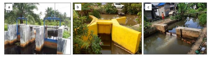
**Figure 5.** Types of water gates: (**a**) flapped water gate, (**b**) swaying water gate, (**c**) stoplog water gate. Photo by Author/Khairil Anwar.
