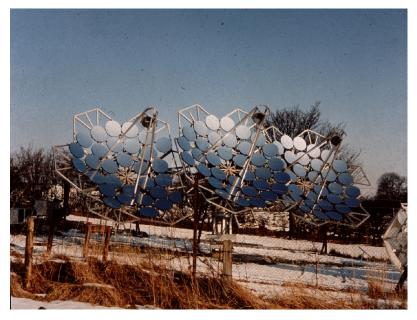
**Figure 3.** The Durham Mark III telescope under construction in Durham, with about 75% of the mirrors in situ. Note the snow on the ground! It is also possible to see the edge of the Mark II telescope at the bottom right, which was rebuilt in Durham for test purposes.
