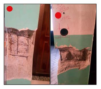
**Figure 5.** Column damages of a building to be demolished. Photos were provided by the study participant upon request of the authors. The intensity value provided by the participant was "Strong".
