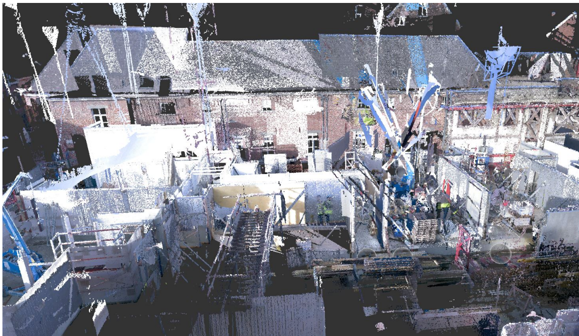
(b) Point cloud captured by Terrestrial laser scanners
