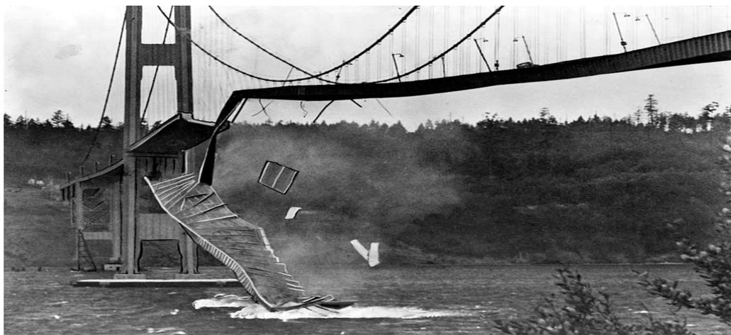
**Figure 1.** Collapse of Tacoma Narrows Bridge (1940) (Source: Wikipedia).
