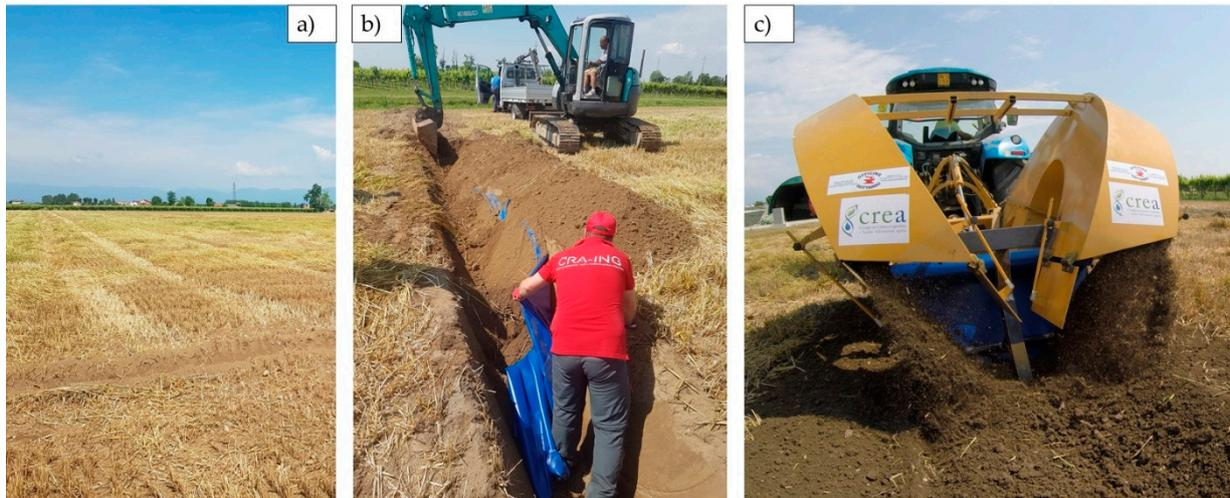
**Figure 4.** Views of (a) the field before building the SWRS, (b) removal of the SWRS using the excavator, and (c) SWRS machinery at work.
