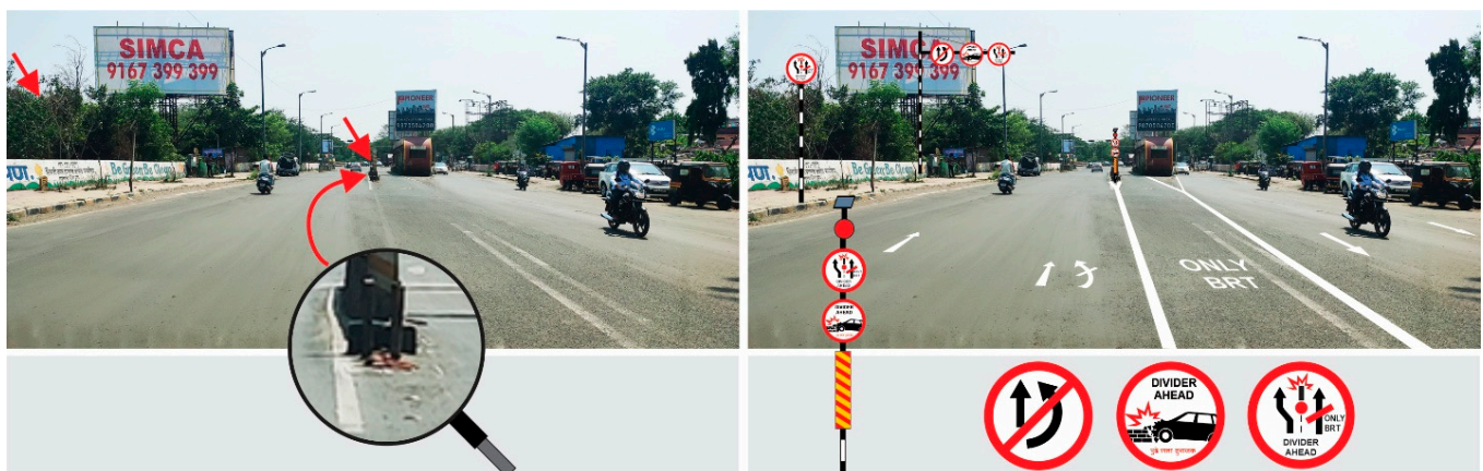
Figure 5. The BRT Lane separates the local bus lane from the main lane.
