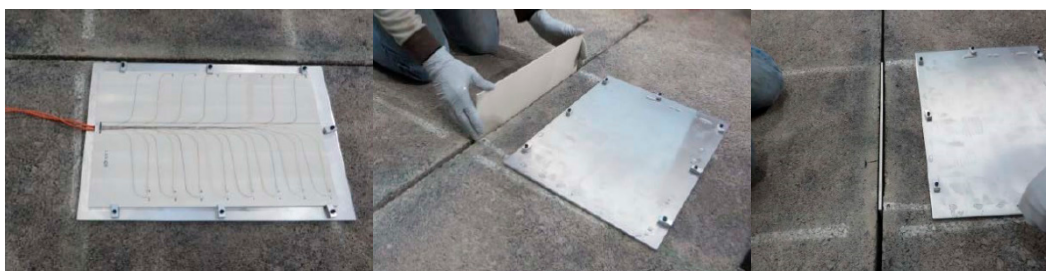
Figure 5. Instrumented plate installation at the Federal Aviation Administration (FAA) National Airport Pavement Test Facility (NAPTF) in Atlantic City, New Jersey, USA (figures are reproduced from Garg et al. [45]).
