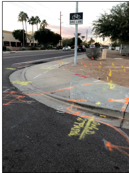
Figure 1. An example of using spray paint and flags to reflect the location of utilities.
