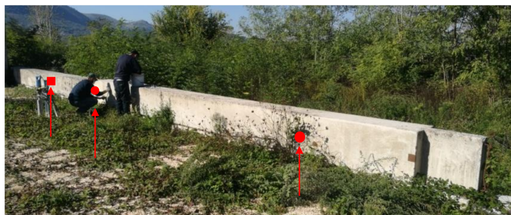
Figure 1. Precast RC squared column “C”; red circles show the location of coring sites; the red square shows the location of the extraction site of the parallelepiped-shaped diamond-cut sample.
