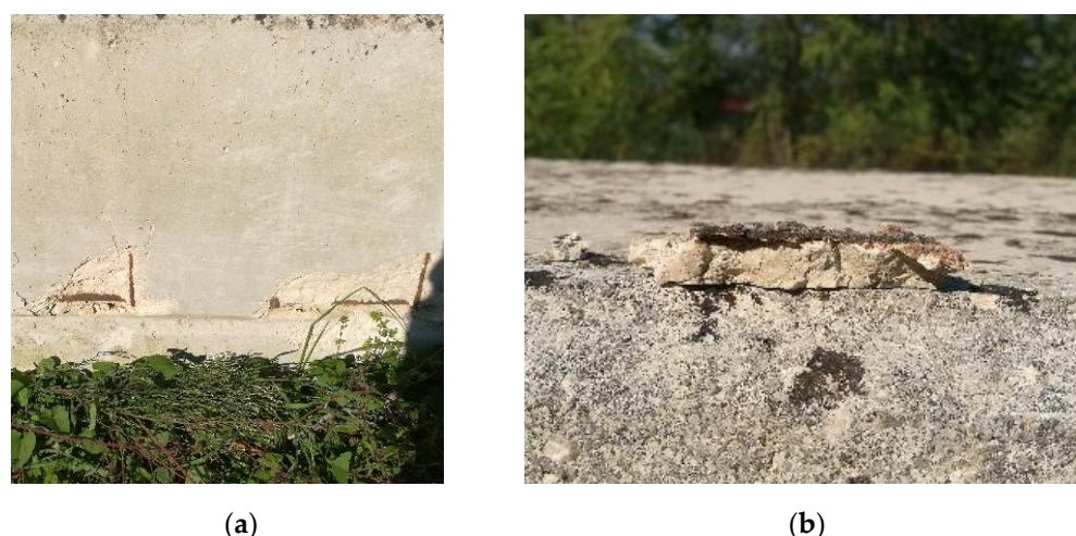
Figure 4. Spalling in column C after struck by hammer (a), detached cover due to hammer strike (b).
