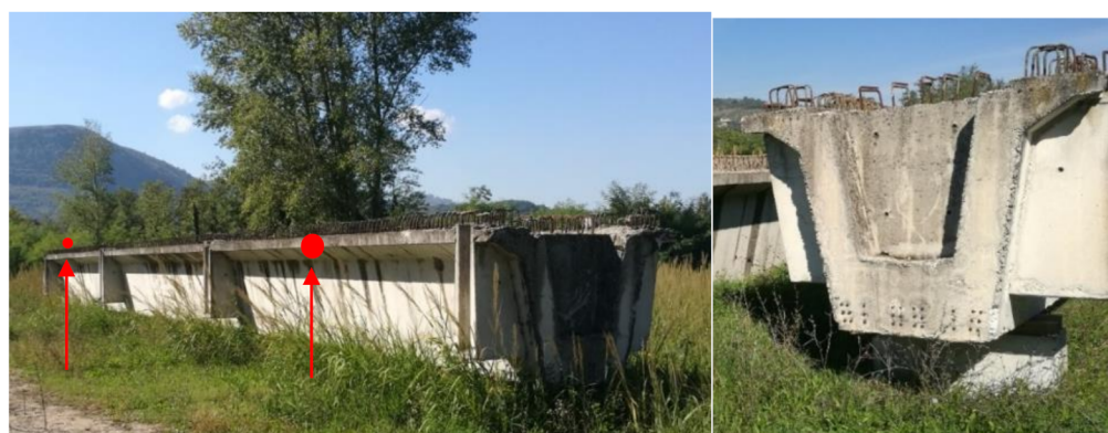
Figure 2. Prestressed RC omega-beam “B1”; red circles show the location of coring sites.
