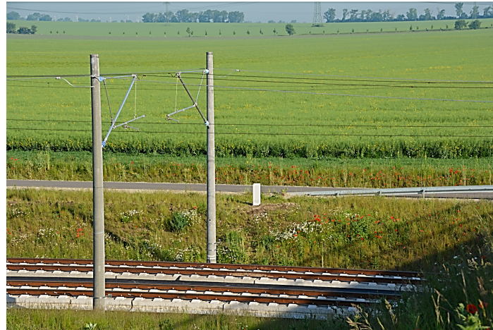
Figure 1. The catenary pole system for high-speed rail routes.
