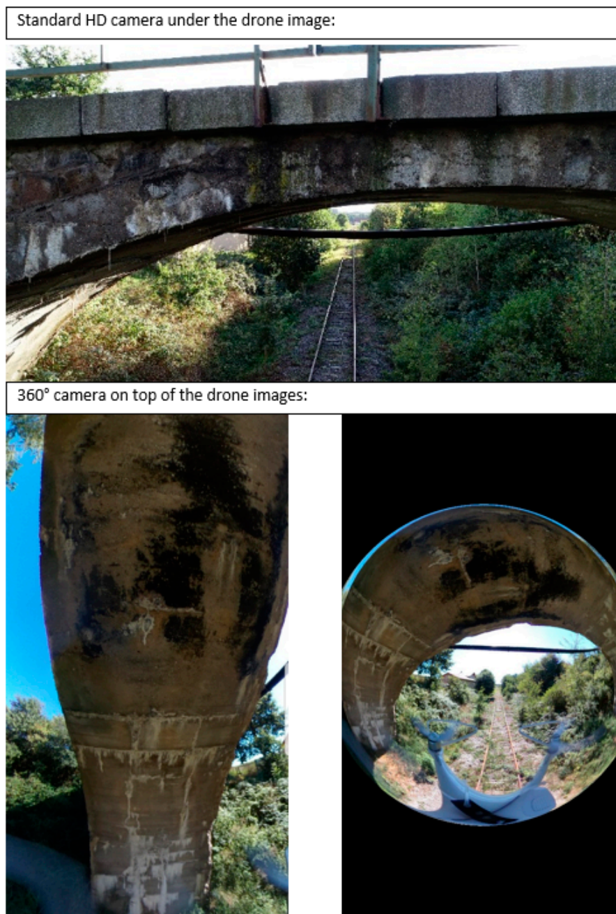
Figure 12. Comparison of the HD and 360° camera images of the arch bridge ceiling.
