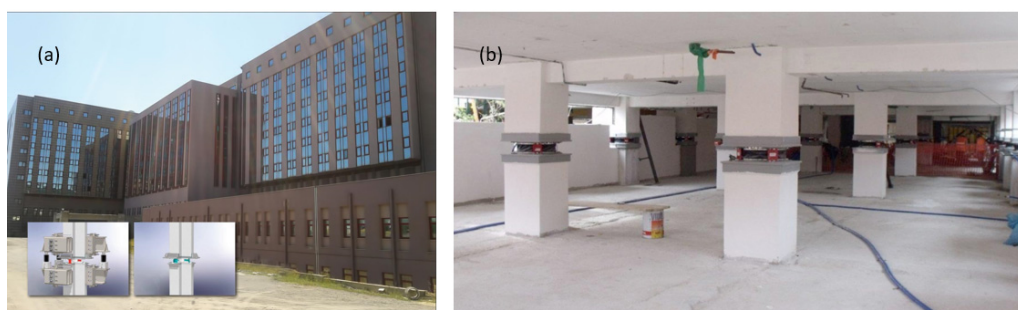
Figure 35. (a) Marmara University Prof. Dr. Asaf Ataseven Hospital and retrofitting procedure (b) Isolation floor of the hospital (Courtesy of Freysaş).
