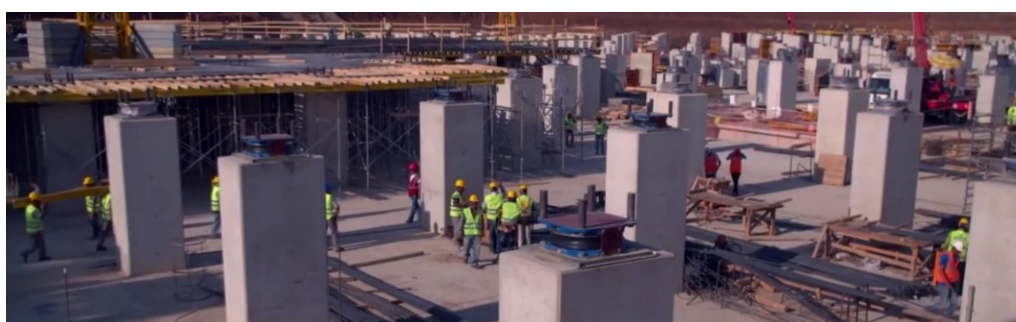
Figure 34. Installation of multi-surface curved surface friction sliders (TFP) for Adana City Hospital (Courtesy of Rönesans Construction Inc., Adana, Turkey).
