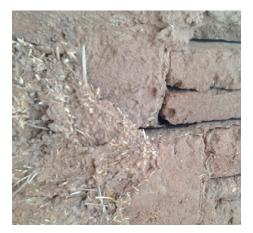
**Figure 7.** Lijiashan Village in Shanxi Province (China). Mud bricks made of the earth of Loess (by F.F. and L.L., 2017).
