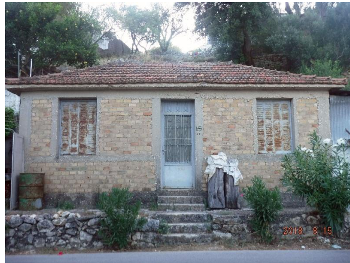
Figure 7. Confined masonry one-storey house in Pastra, with fired-clay bricks, in present condition.
