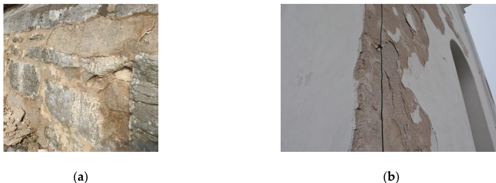
Figure 17. Spalling of lime mortar due to ice formation: (a) When lime mortar freezes and spalls off it leaves a characteristic flake-shaped pattern; (b) each separate render layer spalled off is caused by freezing temperatures in a lean lime render saturated with water.
