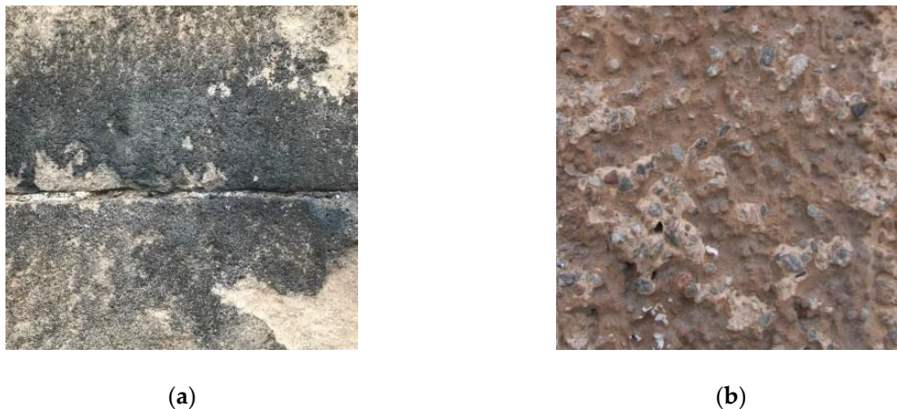
Figure 6. (a) Black crust is usually seen when sulphur has reacted with lime on the surface of calcareous rock or lime render and lime wash; (b) a close-up of a coloured lime cement mortar where the surface has transformed into gypsum. This causes the surface to appear to be very dirty. The original colour of the lime cement mortar can still be observed.
