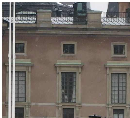
Figure 7. Stockholm Castle showing a coloured lime cement render. As sulphur-containing air causes the formation of gypsum, this usually shows clearly where the rain impinges on a façade. As gypsum is highly soluble in water, the damage is greatest on surfaces sheltered from rain.
