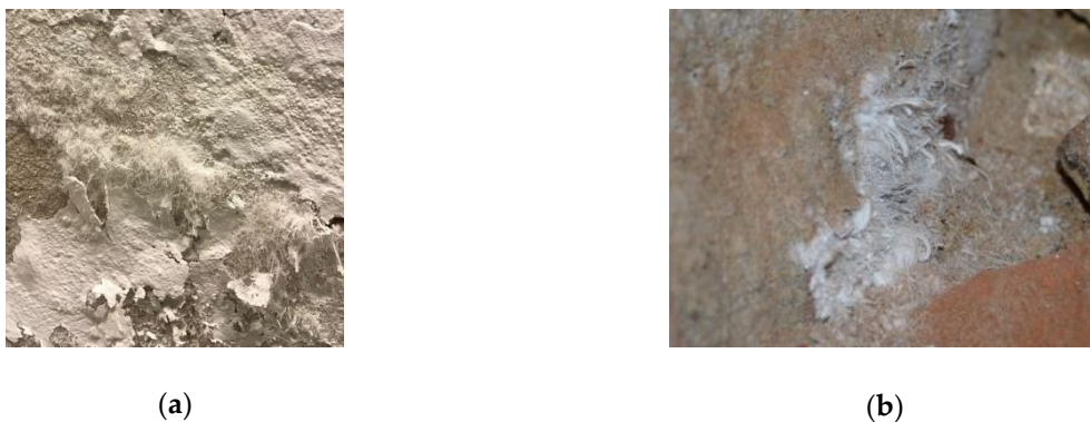
Figure 9. Examples of halite crystals that formed in basements where food had been stored: (a) Halite crystals on a brick wall; (b) halite crystals grow from a surface, forming both compact crystals and long strands.
