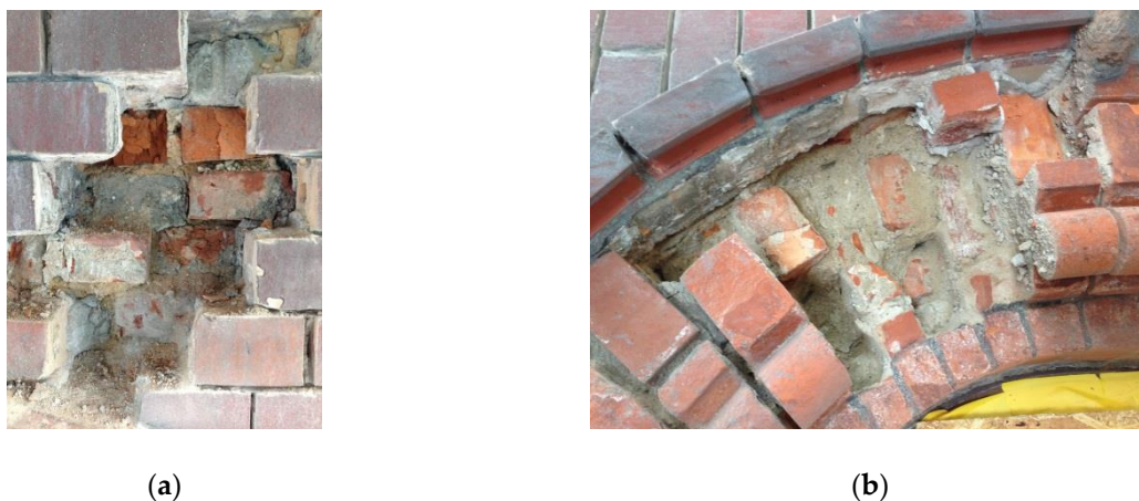
Figure 21. (a) Neo-Gothic masonry where accumulated moisture inside the masonry has caused “masonry rot”; (b) the bricks have frozen and split, while the lime mortar has assumed the character and characteristics of wet sand.
