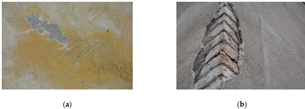
Figure 14. Calcite crystallization and recrystallization: (a) A thick, glassy film of calcite on the external surface of a lime wash. The calcite film prevents new lime wash from attaching, causing the lime wash to spall off when freezing; (b) the surface of a porous lime render restored in the 1970s has changed colour due to some recrystallization.
