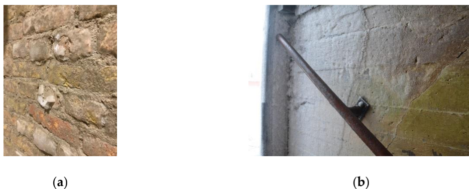
Figure 16. Ice crystal formation on masonry: (a) Ice crystals cover the entire inside of a brick tower on a cold winter's day. Here, the ice crystals have formed an armour-like layer of ice as well as some filiform crystals of approx. 2 cm; (b) an example from a basement where a thick layer of porous ice crystals covers the internal concrete surface. This phenomenon can be observed when porous materials saturated with water are exposed to frost.
