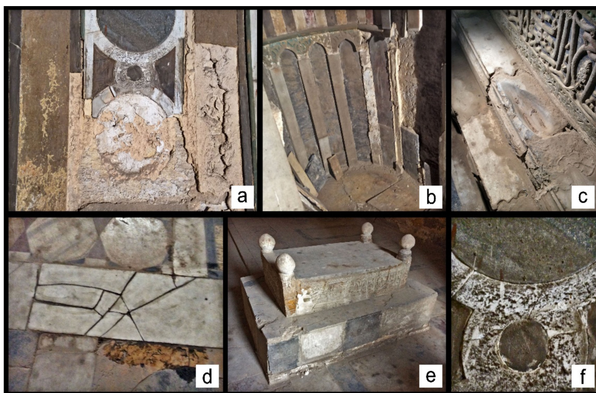
Figure 4. Different forms of deterioration in the northern mausoleum; (a) loss of material, granular disintegration, discoloration; (b) detachment of slabs; (c) fractures, erosion; (d) fractures; (e) loss of material, fractures, erosion; (f) organic staining, efflorescence.
