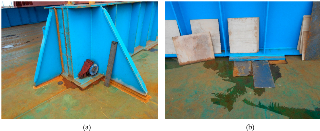
Figure 9. (a) Longitudinal and transverse brackets; (b) Thin metal ready to be placed below the central bearing plate.
