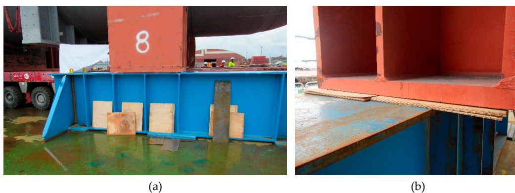
Figure 10. (a) Cradle in the position just over the three stiffenings. The two stiffenings of the beam-ends aligned with the bearing plates. (b) Plywood as dunnage placed in the void space between the cradle and the grillage beam.
