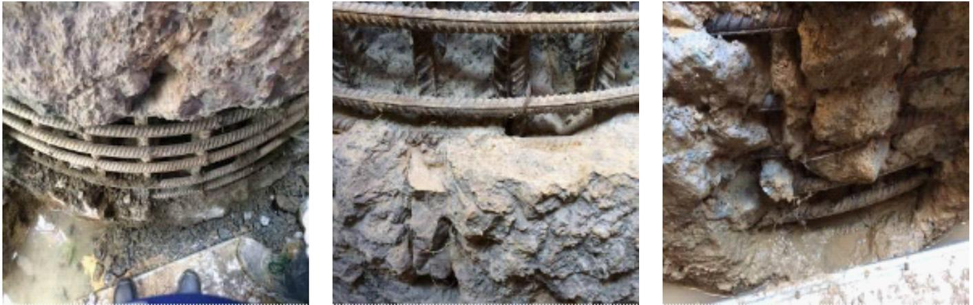
**Figure 1.** Faults in the cover zone due to incomplete filling as a possible result of highly reinforced cages or insufficient workability, i.e., rheological behaviour of the concrete (Bauer Spezialtiefbau GmbH).
