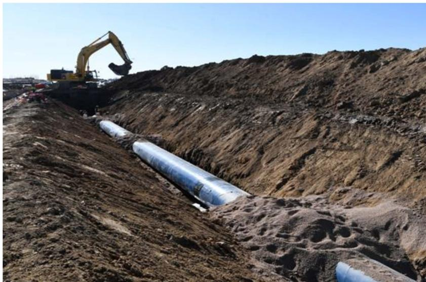
**Figure 1.** A gas pipeline being buried in construction.
