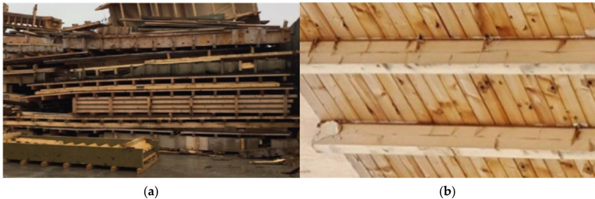
**Figure 3.** (a) Depot of timber formwork for reuse. (b) Reused formwork [29].
