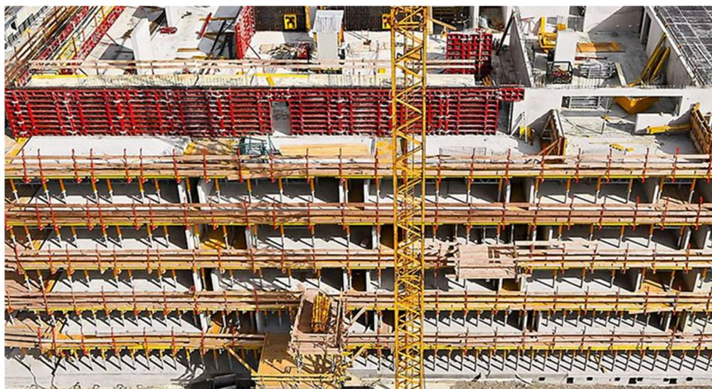
**Figure 2.** Cast-in-place construction of a multi-story concrete structure with horizontal and vertical formwork and supporting shores.
