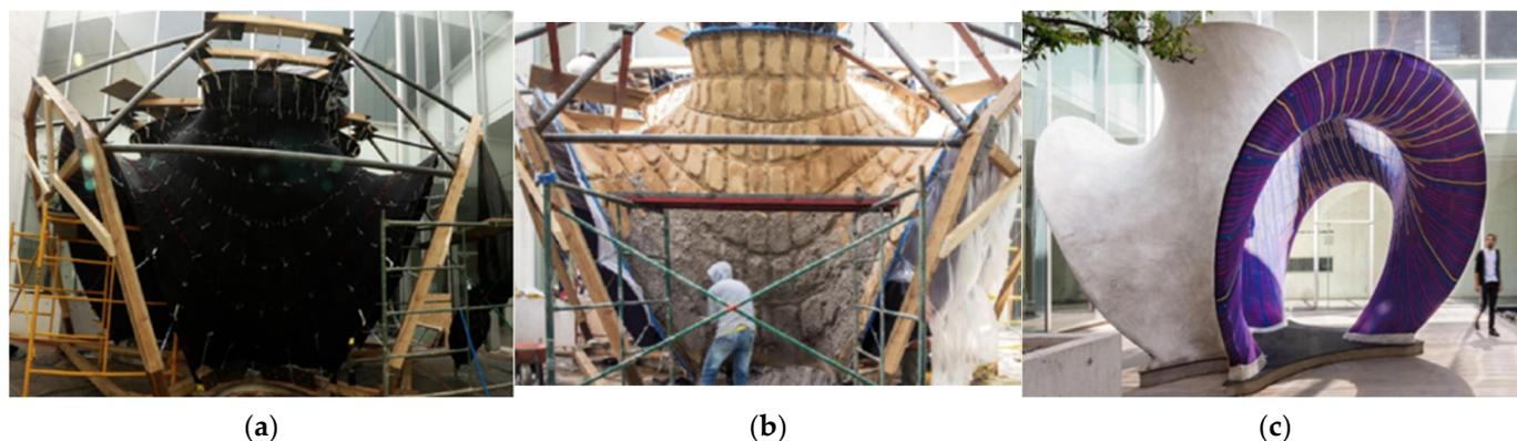
**Figure 4.** The KnitCandela concrete shell [156]. (a) Knitted textile formwork (photo: Maria Verhulst); (b) first layer of concrete (photo: Mariana Popescu); (c) finished concrete shell with textile interior (photo: Angelica Ibarra).
