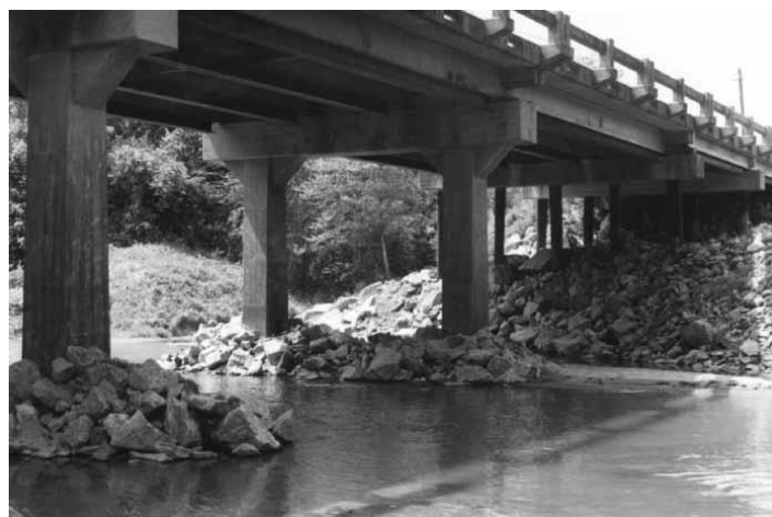
Figure 4. Riprap used to protect bridge piers from scour [23].
