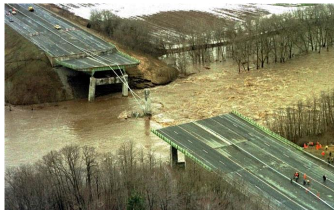
Figure 1. Schoharie Creek bridge collapse in 1987 after the scouring of one of its bridge piers' foundations [6].
