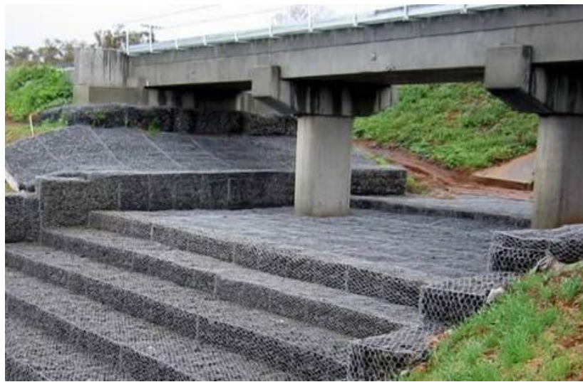
Figure 6. Example of a stepped gabion mattress formation to prevent bridge pier scour [34].
