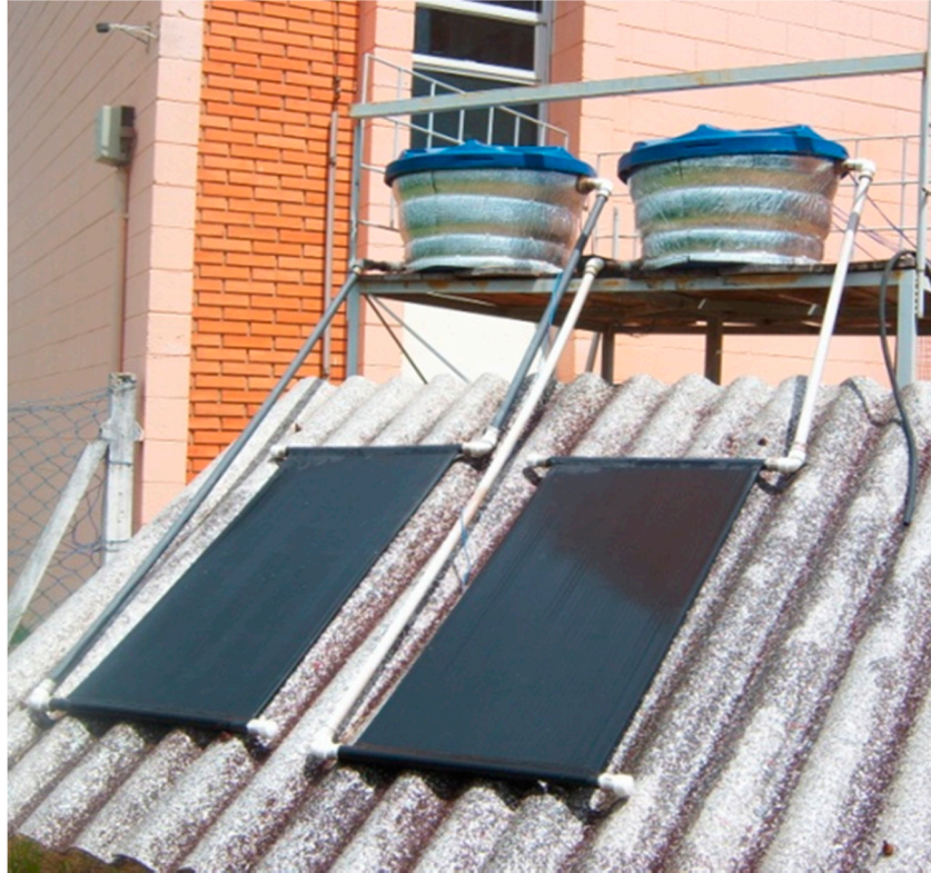
Figure 2. Two low-cost solar heating systems assembled (100 L each): PVC solar collector and hot water reservoir with thermal insulation (polymeric coating) outside the tank.
